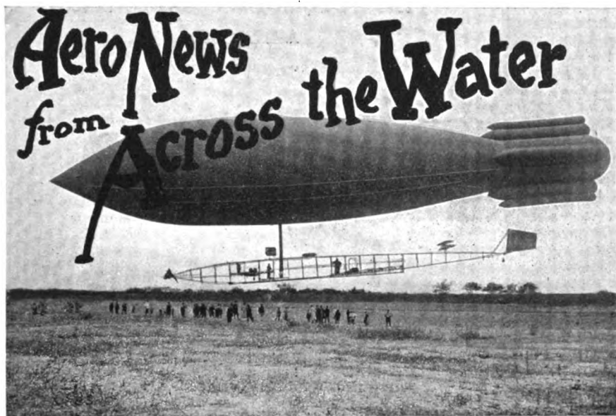
VILLE DE PARIS BEGINNING WORK AGAIN AFTER ITS ACCIDENT.
